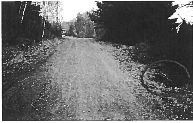
Figure 2: Erosion at culvert indicated by red circle
